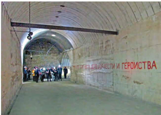
High arched tunnel in Objekt B, showing precast concrete reinforcements. The Russian inscription is probably from more recent filming in the complex
